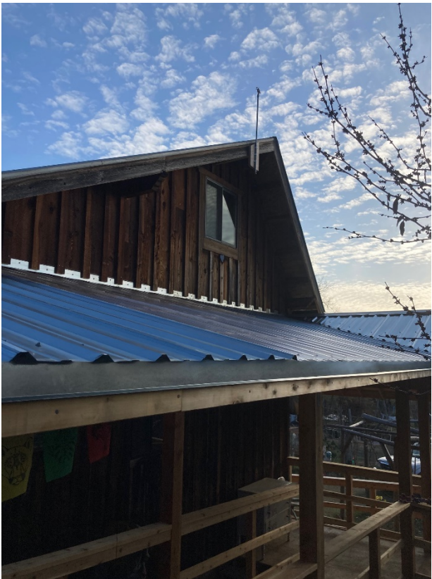
Figure 4 a) rainbird-type sprinkler affixed near house roof peak has swivel connector for \frac{3}{4} " GHT (garden hose) connector for use with \frac{3}{4} " "p-line" firehose. b) similar sprinkler on fencepost near house and outbuildings; bottom of standpipe tees into fitting for 1" firehose. Pipes must be metal, not plastic!
