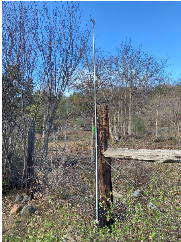
Figure 4 a) rainbird-type sprinkler affixed near house roof peak has swivel connector for \frac{3}{4} " GHT (garden hose) connector for use with \frac{3}{4} " "p-line" firehose. b) similar sprinkler on fencepost near house and outbuildings; bottom of standpipe tees into fitting for 1" firehose. Pipes must be metal, not plastic!
